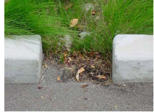
Curb cutouts deliver runoff from a parking lot to a vegetated swale. Vegetation must be lower than pavement to prevent clogging and sediment build-up at the curb. Photo: City of Fremont
