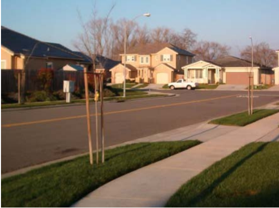
Divided sidewalks in a new residential subdivision are one form of disconnected pavement. Photo: ECorp Consulting
