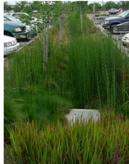
Alternative vegetation is encouraged but is subject to approval of local permitting agency. Parking lot swale at Elk Grove Marketplace, Elk Grove, CA. Photo: CKB Environmental
