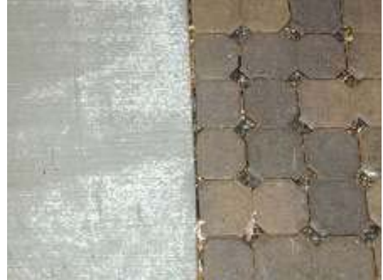
A water barrier or interceptor drain will be required between regular load-bearing pavement/streets and porous pavement materials. Photo: City of Portland
