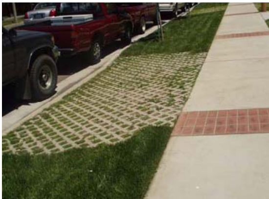
Use of reinforced grass pavement (“grasscrete”) allows for pedestrian access without vegetation damage and reduces runoff through infiltration. Photo: Alameda Countywide Clean Water Program.
