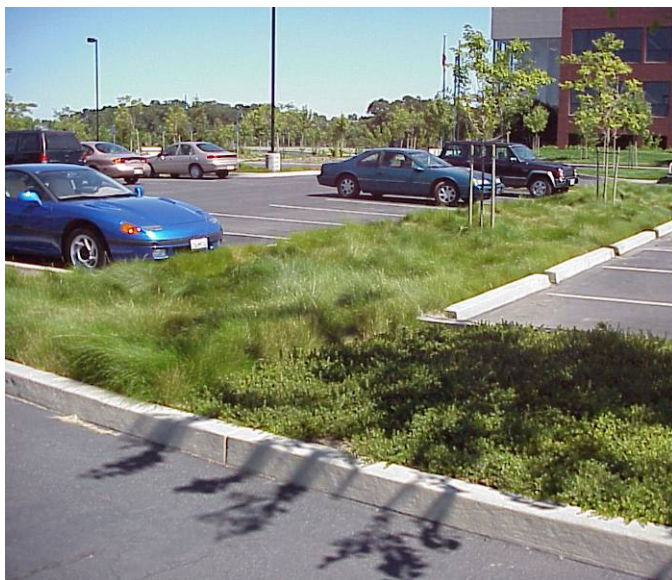
Vegetated Swale Planted with Native Clump Grasses (note that trees as shown are now discouraged; locate outside of flowline), U.S. Farm Bureau, Sacramento. Photo: City of Sacramento
